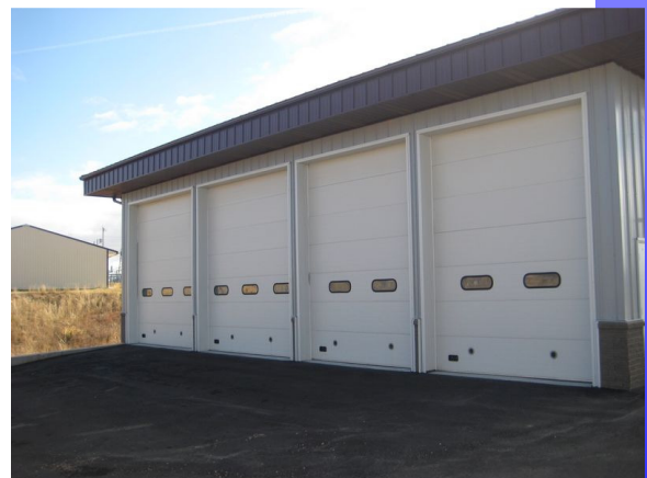
14' overheads on 2 nd building
