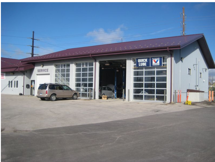
12' overheads on main Building
